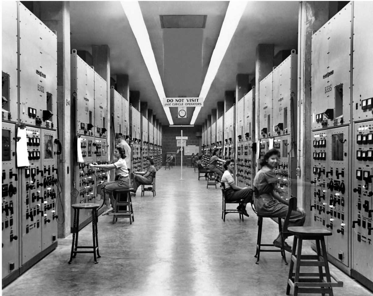
Image 3: Calutron operators at the Y-12 plant in Oak Ridge monitored indicators and turned dials in response to changing values, not knowing that they were actually aiming streams of uranium ions, much less that they were producing the fuel for a new weapon. Source: Photo by Ed Westcott, 1944 (Department of Energy).
